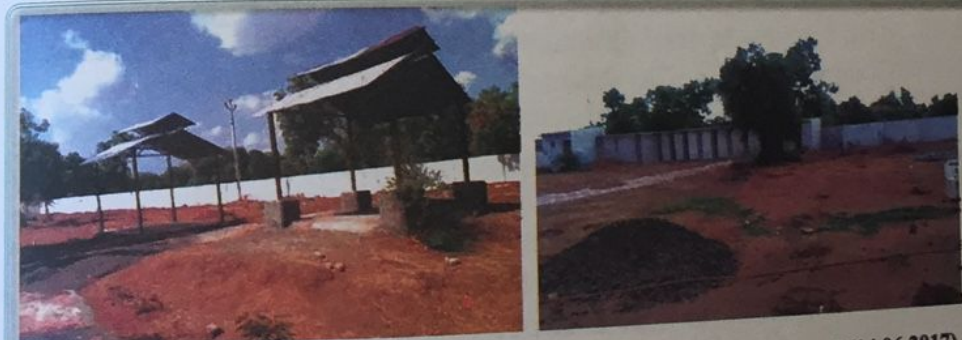
Picture 8: Incomplete construction of crematorium for Kshatriya Samaj (14.06.2017)
