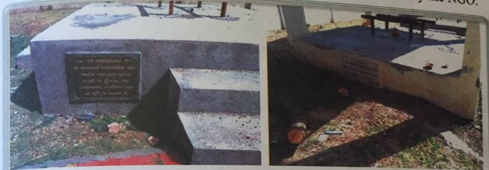
Picture 7: Construction of crematorium for Patel Samaj done by the donors (14.06.2017)
