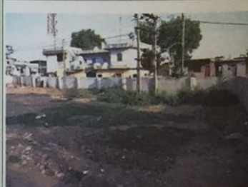
Picture 5: Block paver not laid near Artificial Insemination Centre at Udhel (13.06.2017)
